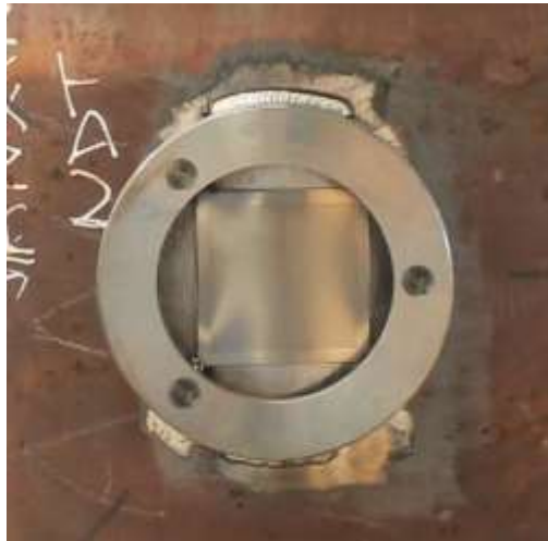
High temperature resistant grid pattern superimposed on P91 pipework.
